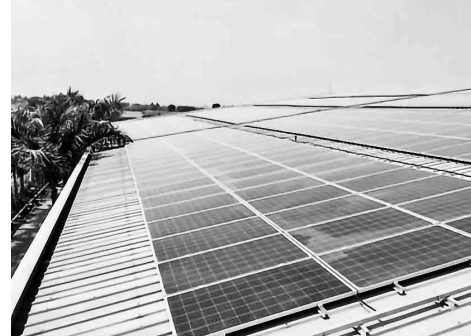
Solar Panel Installation Seco India
